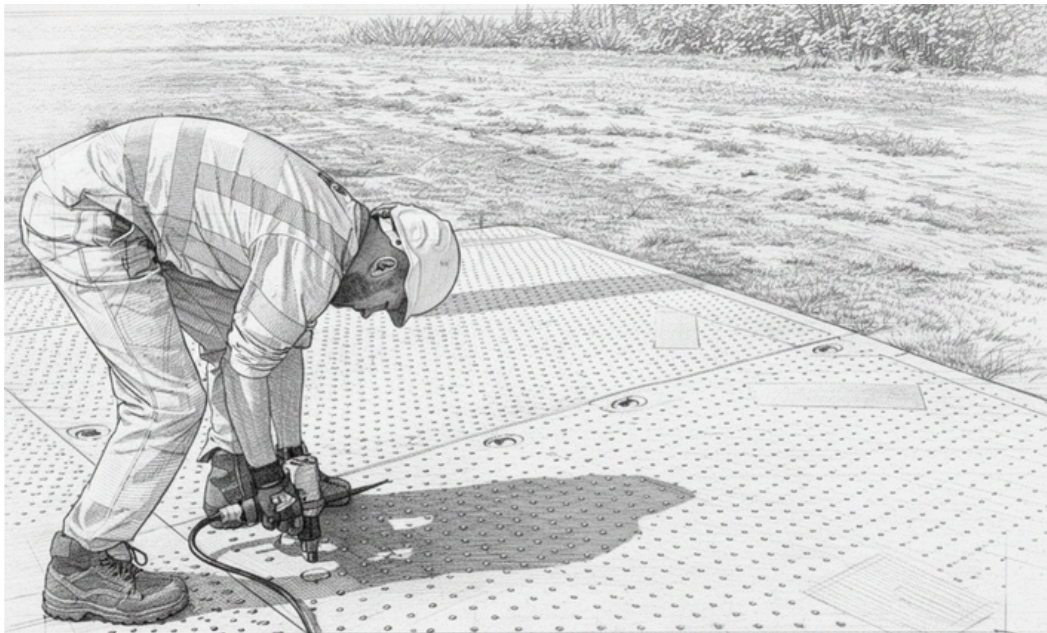
Figure 6m: Tightening a bolt on a terrain
