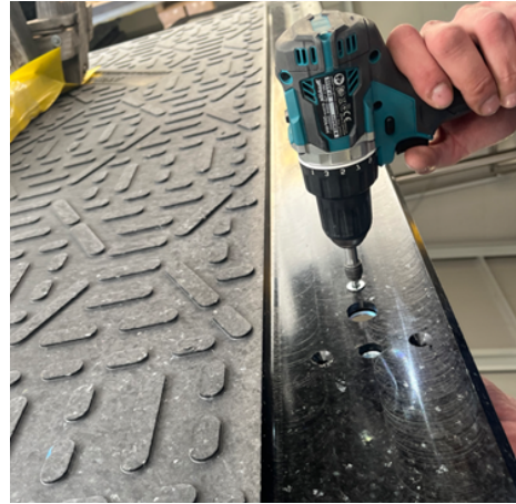
Figure Appendix 3g: Tighten all bolts
