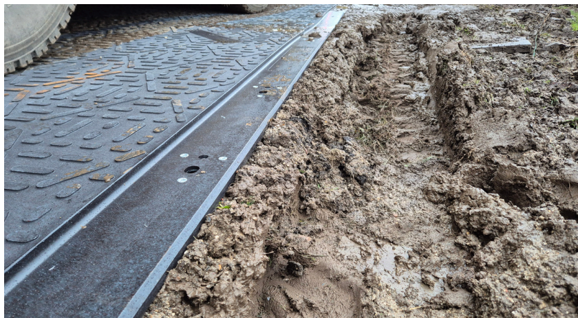
Figure 4k: H-overlap mat in muddy conditions
