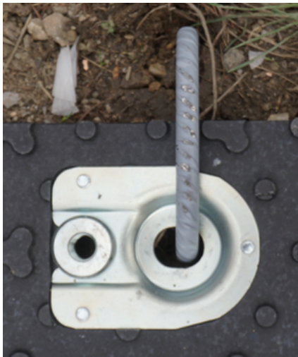
Figure 7e: Hammer the U-pin into the ground
