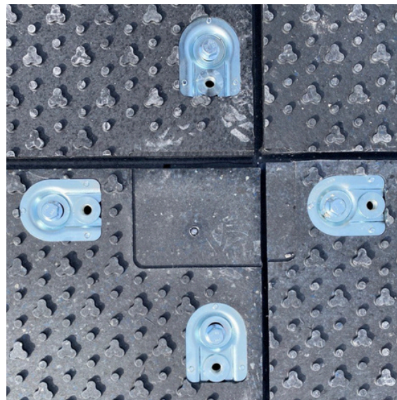
Figure 6o: Properly inserted and fastened bolts
