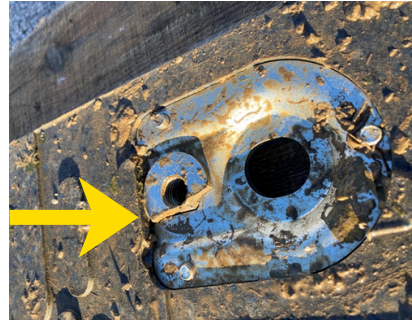
Figure Appendix 3a: Damaged exchangeable nut
