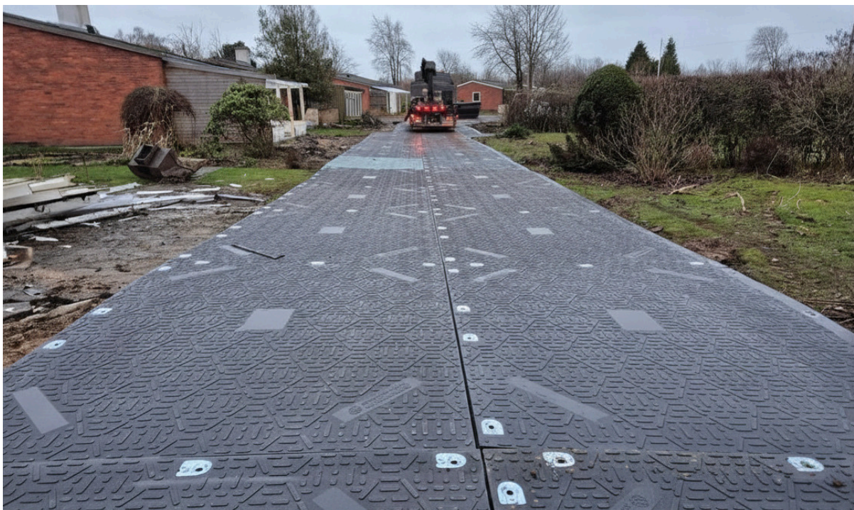
Figure 1: Equipment on Isotrack H-Overlap
