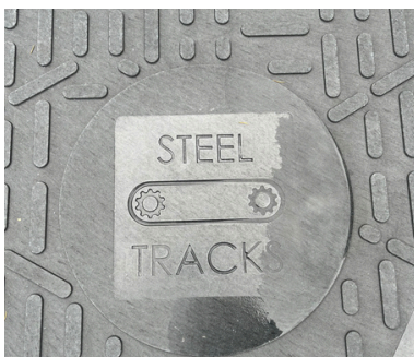
Figure 2b: Surface for Steel Tracked Vehicles
