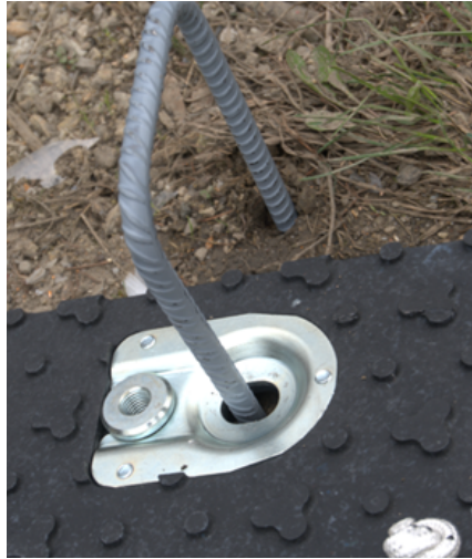
Figure 7d: Position the U-pin in the proper hole
